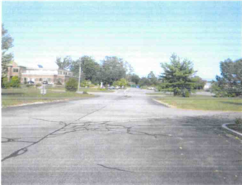
Front Entranceway – New Hampshire Avenue
