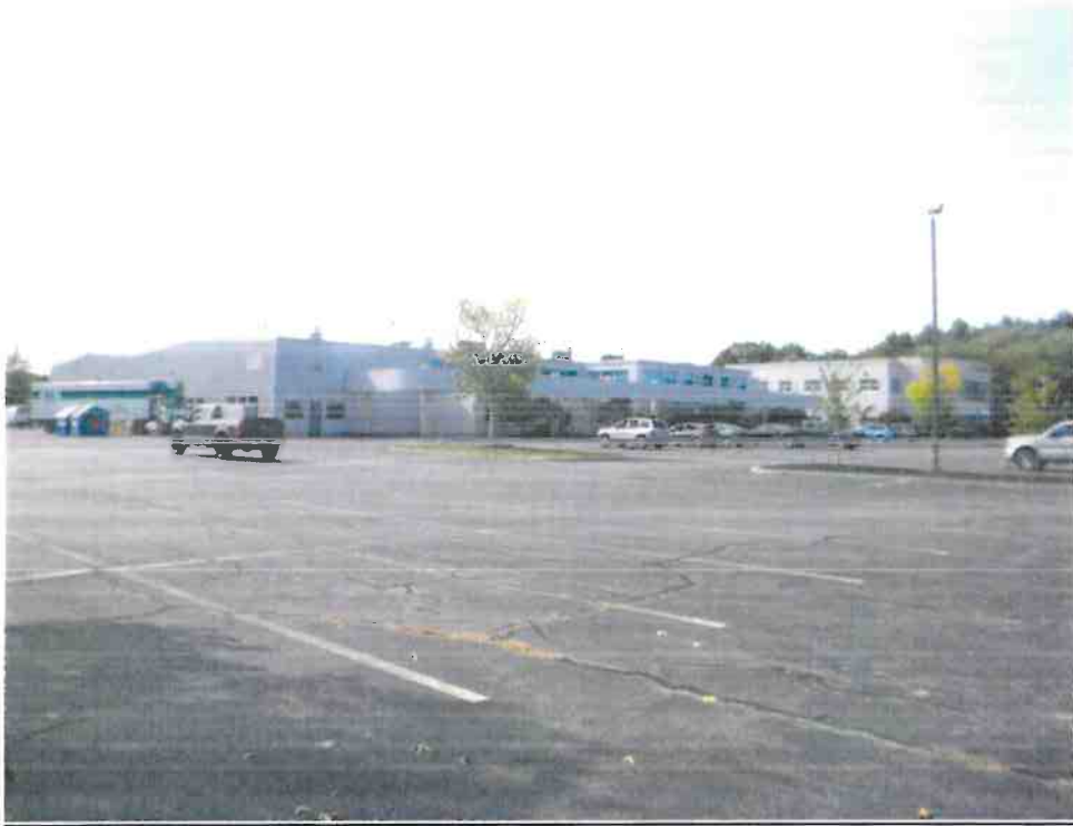
Front of Subject Complex
