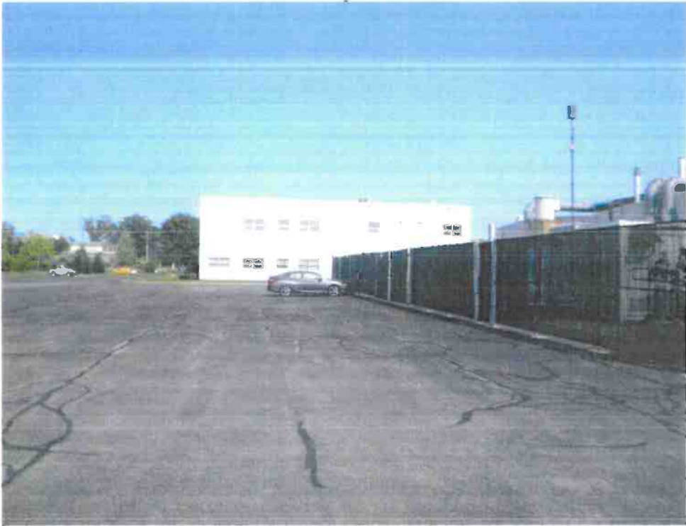
Rear of Subject Section & Office Section
