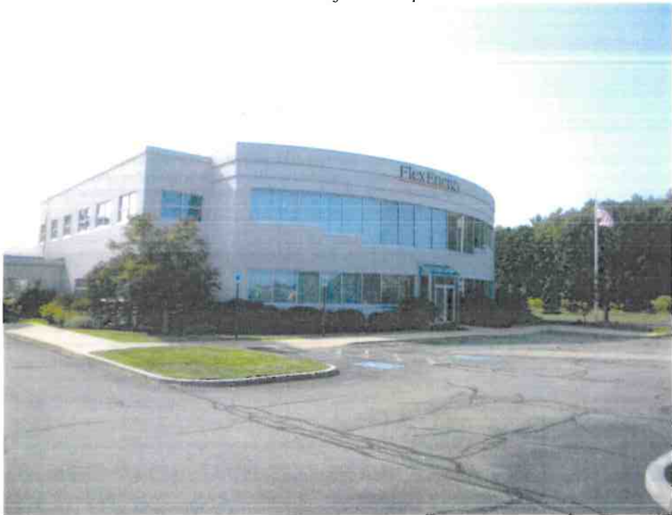
Front of Subject Complex
