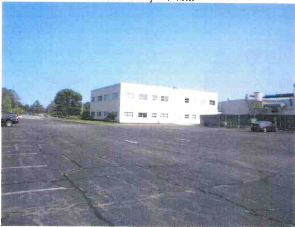
Rear of Office Section
